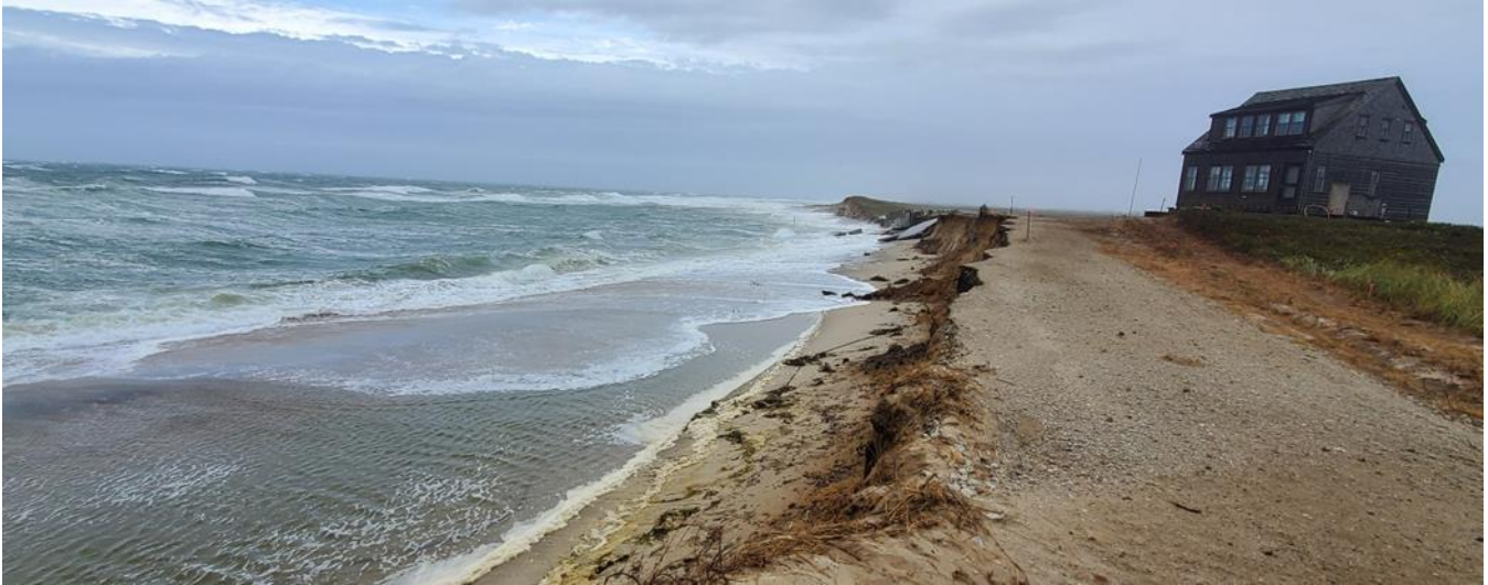
Figure 19. Coastal erosion impacting a private access road, September 2020
