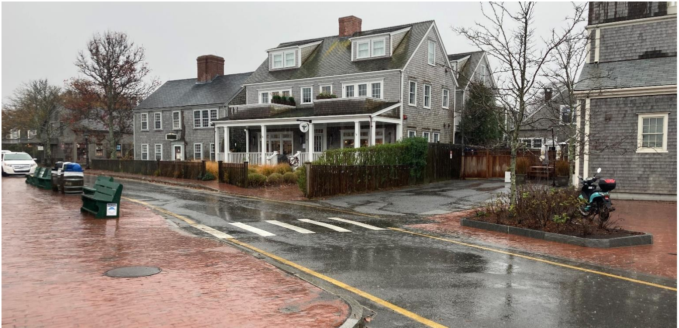
Figure 21. Stormwater flow and ponding in streets in Downtown Nantucket, November 2020
